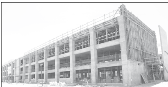
MCRD San Diego's future recruit barracks is expected to be completed spring 2028. Photo by Mario Icarl
